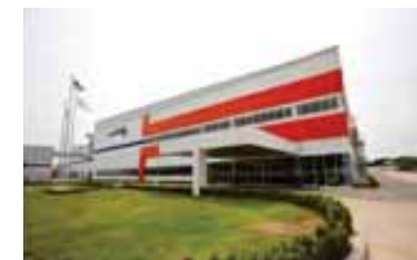
Saha Seiren Factory Kabinburi Industrial Zone, Thailand | 2011
