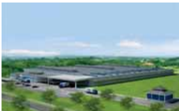
Hino Motors Factory Bukit Indah Industrial Park, Indonesia | 2012
