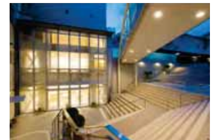
Hosen Gakuen Gym Seismic Strengthening | Tokyo | 2012
