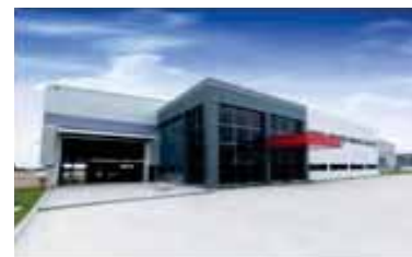
Shinpack Factory Pinthong Industrial Estate, Thailand | 2012
