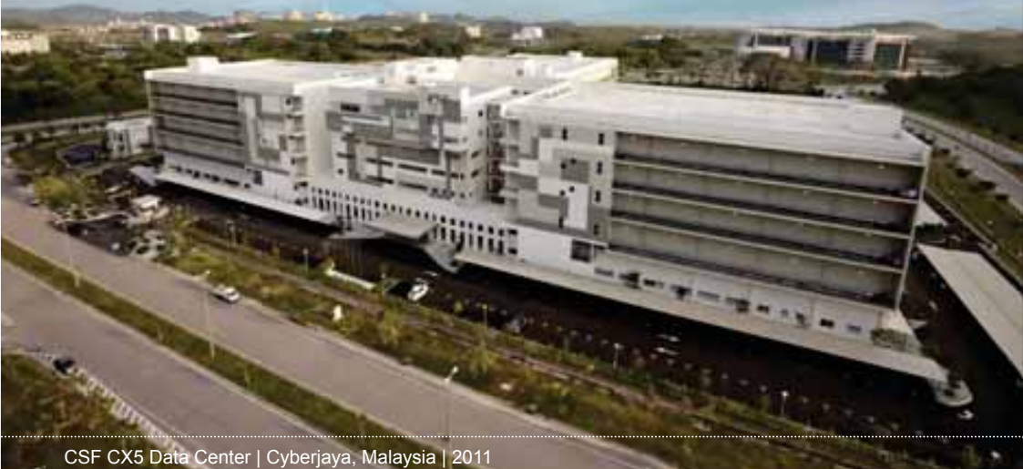
CSF CX5 Data Center | Cyberjaya, Malaysia | 2011
